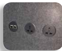
AH Meyer Power & RJ45 Data Point
